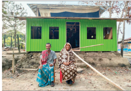
Rehabilitation of a house for delwar hawladar
