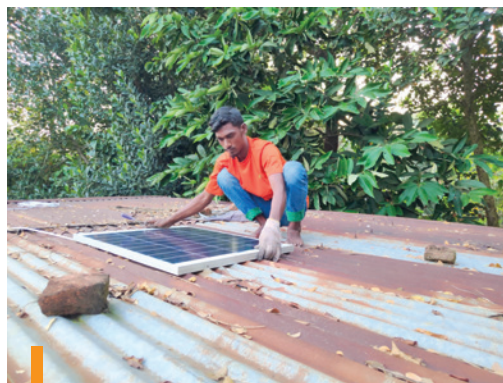
Installing solar panels
